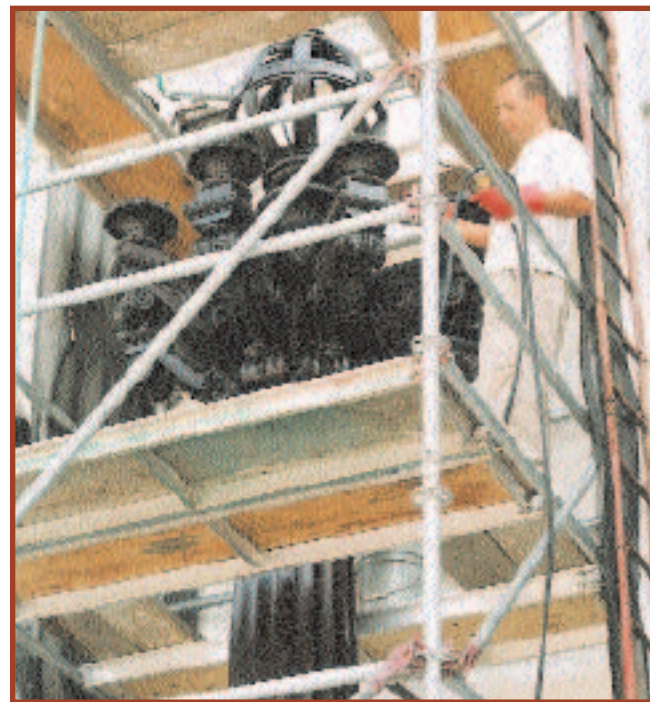
CONSERVATOR APPLYING PATINA TO THE LIGHT STANDARDS LOCATED AT THE CAPITOL'S MAIN ENTRANCE
