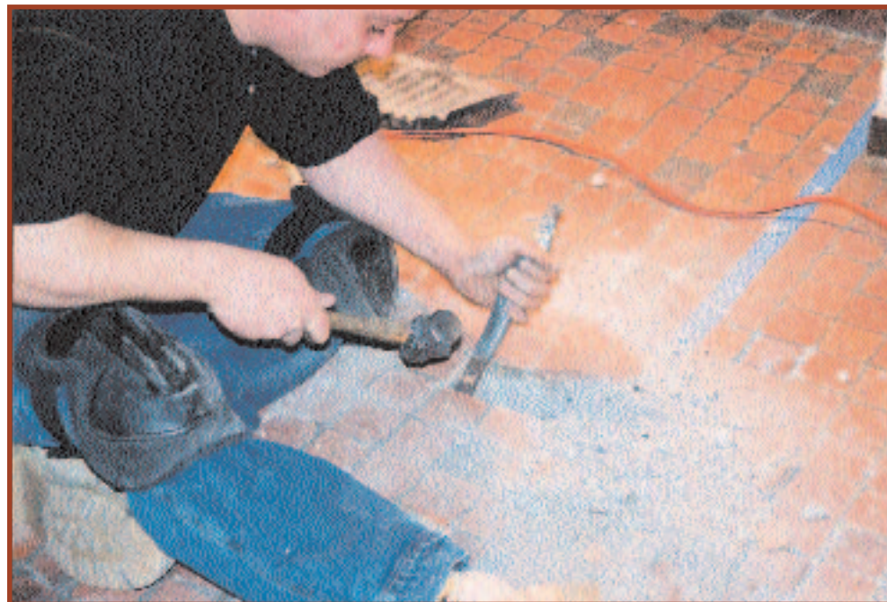
REMOVAL OF INDIVIDUAL WORN TILES USING CHISEL AND HAMMER
