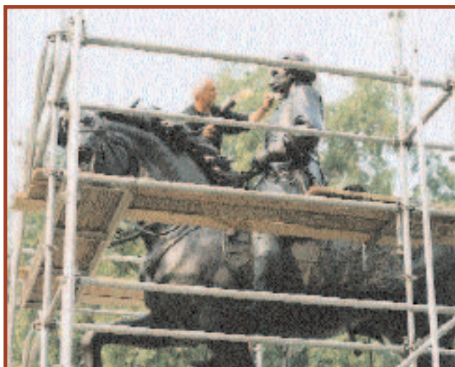
A TINTED HOT WAX IS APPLIED TO THE HARTRANFT MEMORIAL USING A BLOWTORCH
