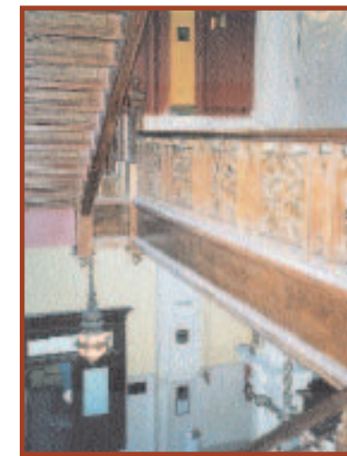
STAIRCASE RESTORATION SENATE FLOORS
