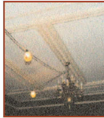
ROOM 462 DURING RESTORATION
