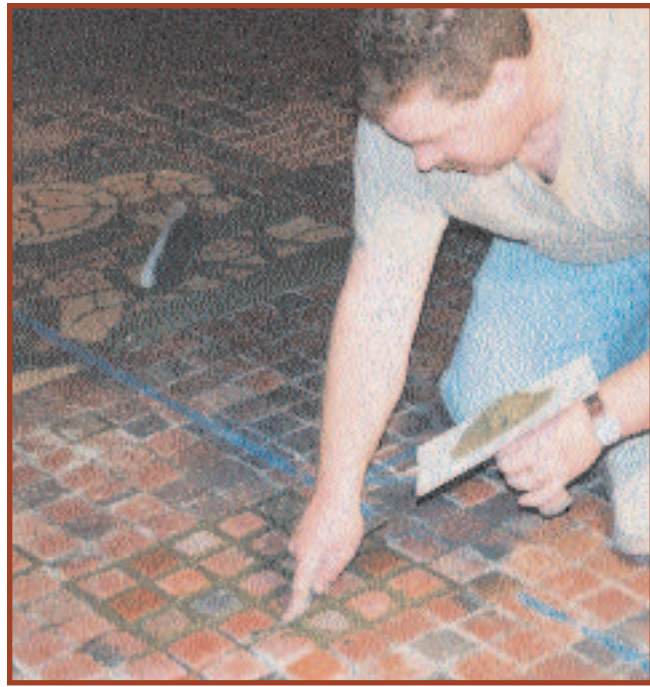
GROUTING IN NEW REPLACEMENT TILES
