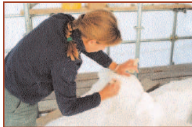
CONSERVATOR REMOVING FAILED GROUT JOINT
