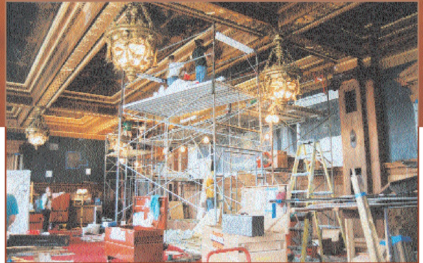
WORK IN PROGRESS...THE COORDINATION OF MULTIPLE TRADES
