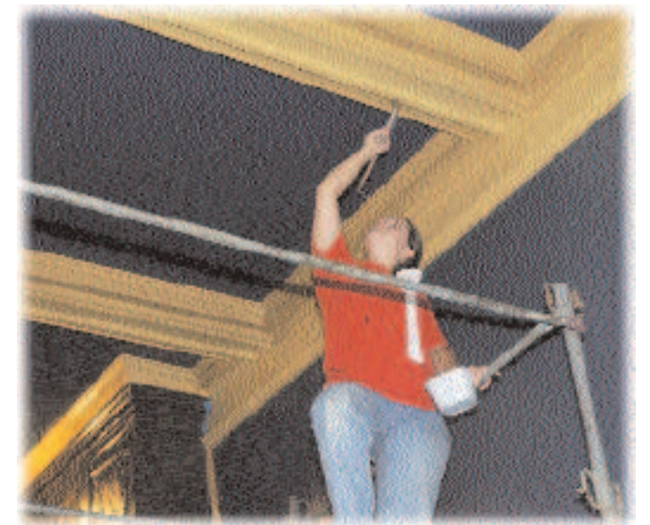
GLAZING UNDERSIDE OF COFFER
