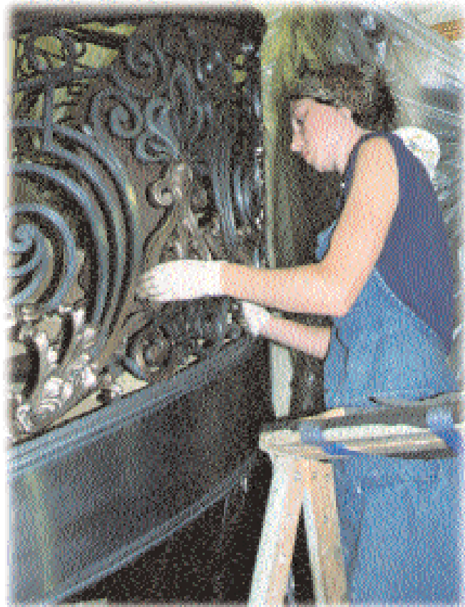
RESTORING BRONZE SPIRAL STAIRCASE
