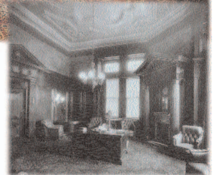
ROOM 238 HISTORIC 1906 PHOTOGRAPH
