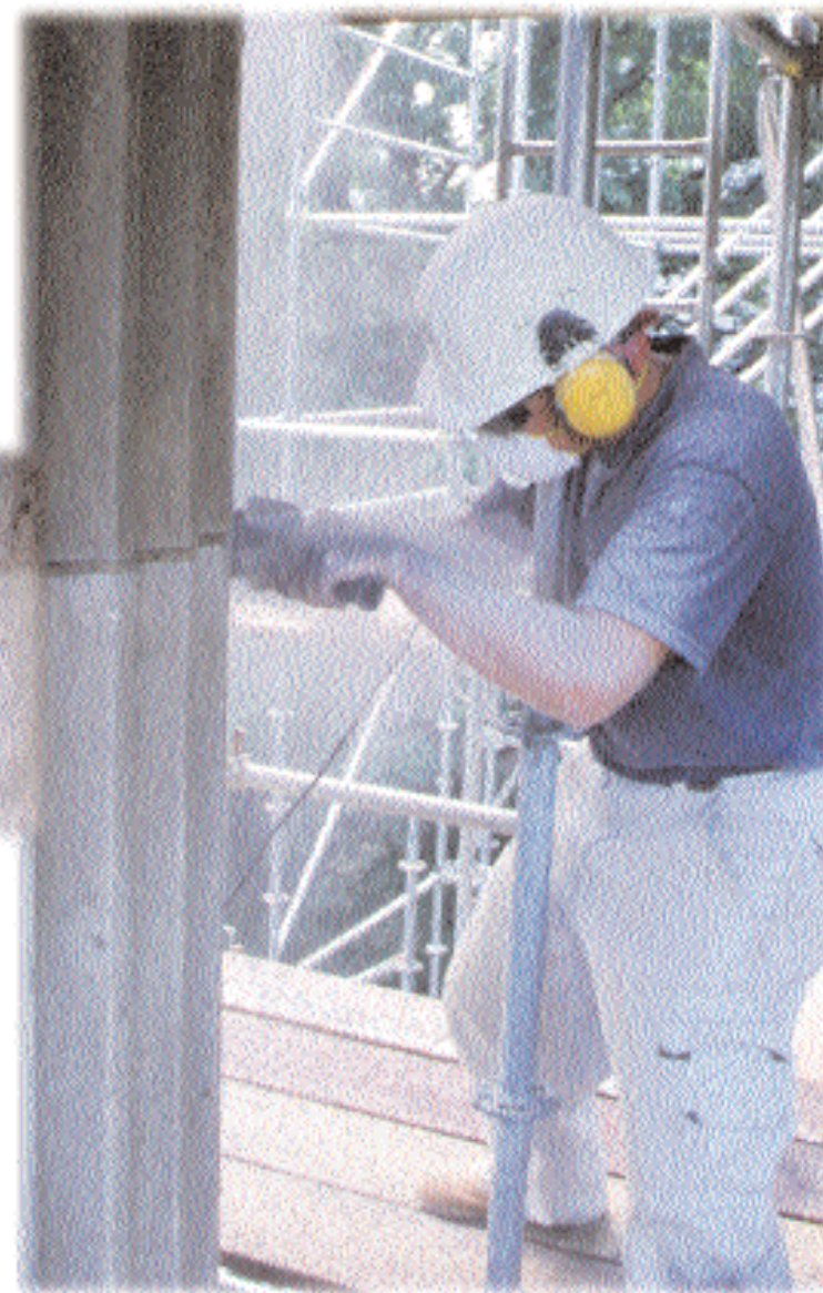
REPAIR OF MORTAR JOINT
