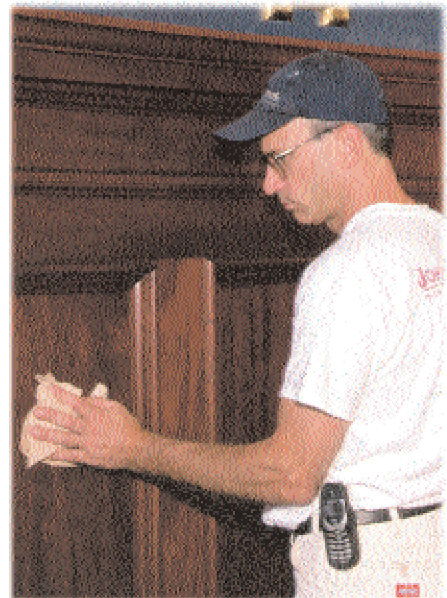
APPLYING STAIN TO WOODWORK
