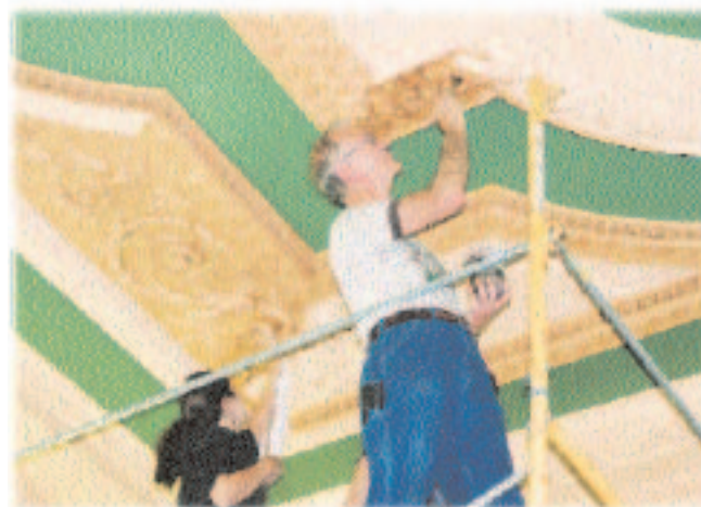
APPLYING GLAZE TO DECORATIVE MOULDING
