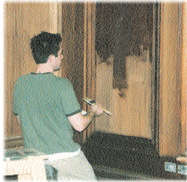
APPLYING WOOD CONDITIONER
