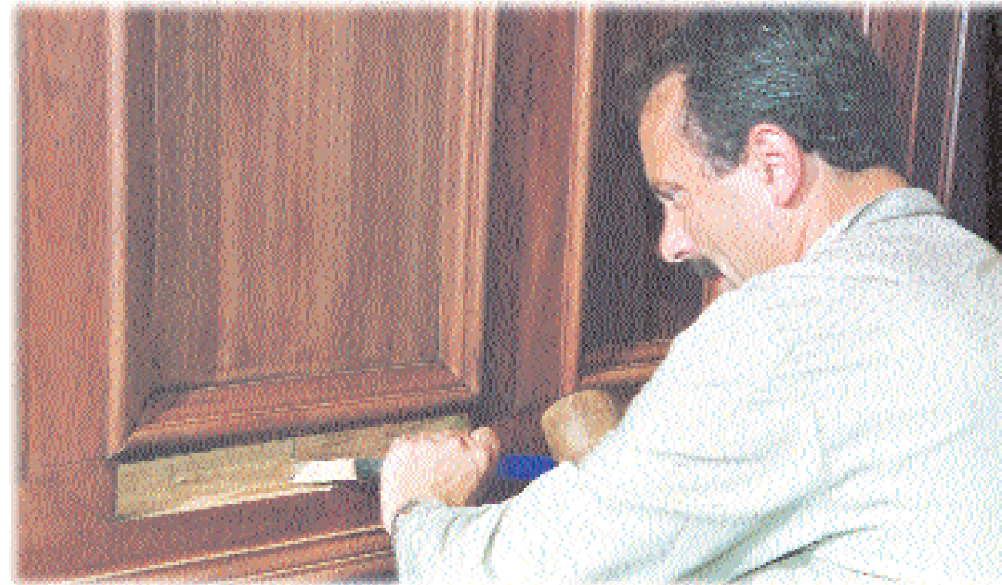
REMOVING VOID AREA FOR INSTALLATION OF DUTCHMAN REPAIR
