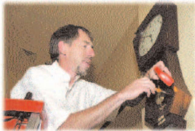
INSTALLING CONSERVED CLOCK
