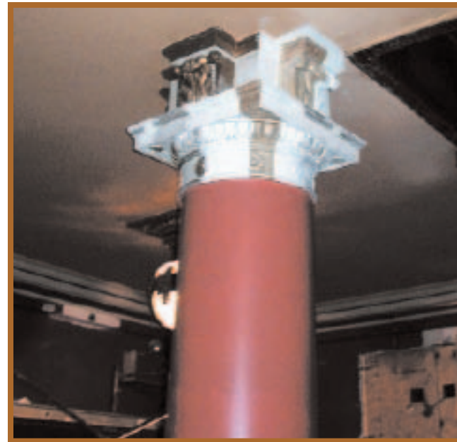
COLUMN PRIOR TO RESTORATION
