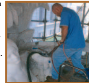
CORE DRILLING ANCHOR HOLES
