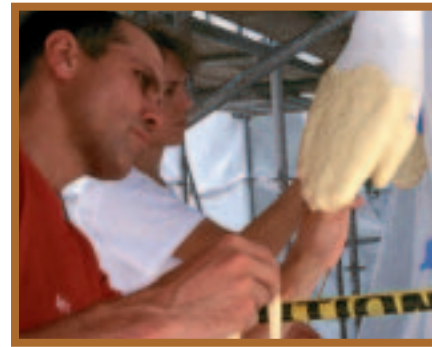
PREPARING SILICONE RUBBER MOLD
