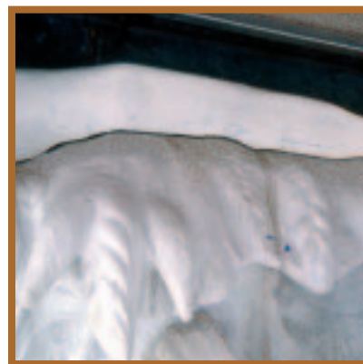
MID-TREATMENT: PERMANENT FIBERGLASS CAP INSTALLATION
