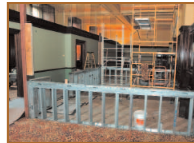
110 SUITE TELLER'S STATION DURING RESTORATION
