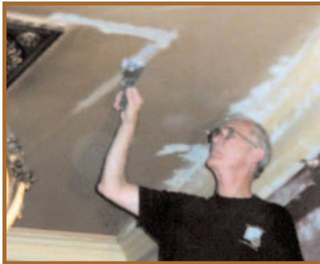
REPAIRING CEILING AND CORNICE
