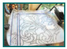
Replacement glass was only installed for areas that contained multiple fractures where safety and integrity were a concern. Fortunately, the
