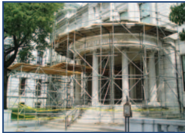
RYAN BUILDING RESTORATION
