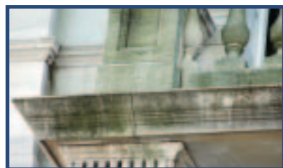
BALCONY BEFORE RESTORATION
