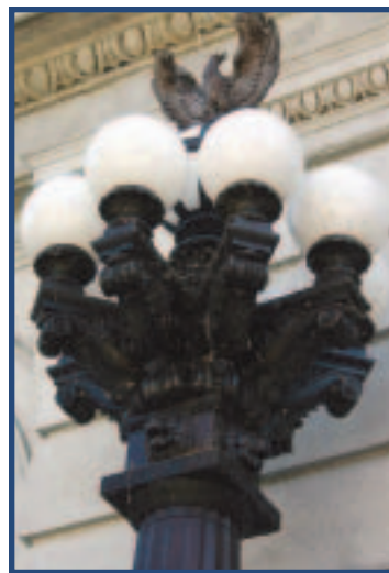
LIGHT STANDARD BEFORE CONSERVATION MAINTENANCE
