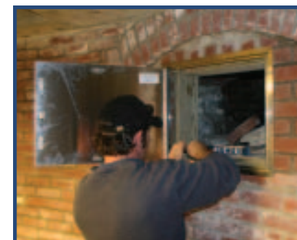
INSTALLING NEW ACCESS PANELS
