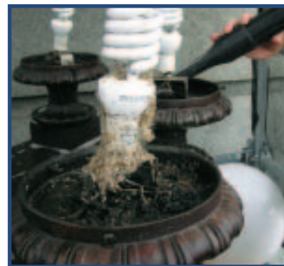
VACUUMING DEBRIS ACCUMULATED INSIDE GLOBES
