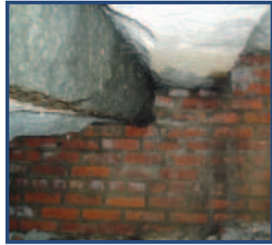
UNDERSIDE VIEW OF STEPS
