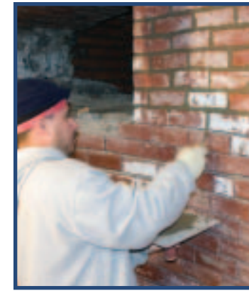
REPOINTING BRICK WALL
