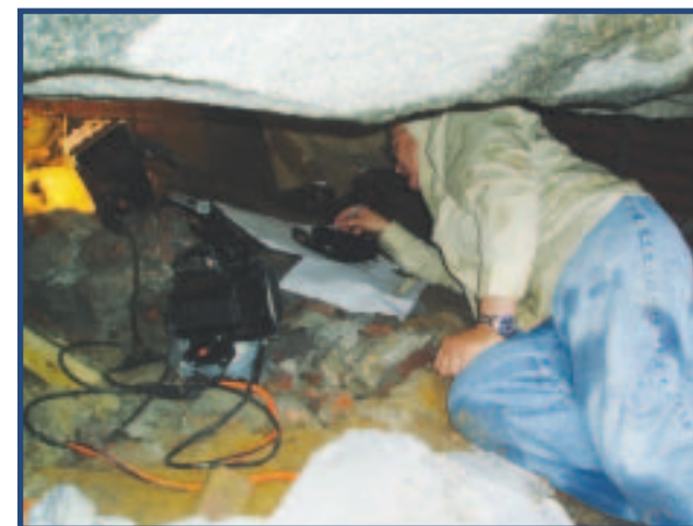
INSPECTION UNDERNEATH STEPS
