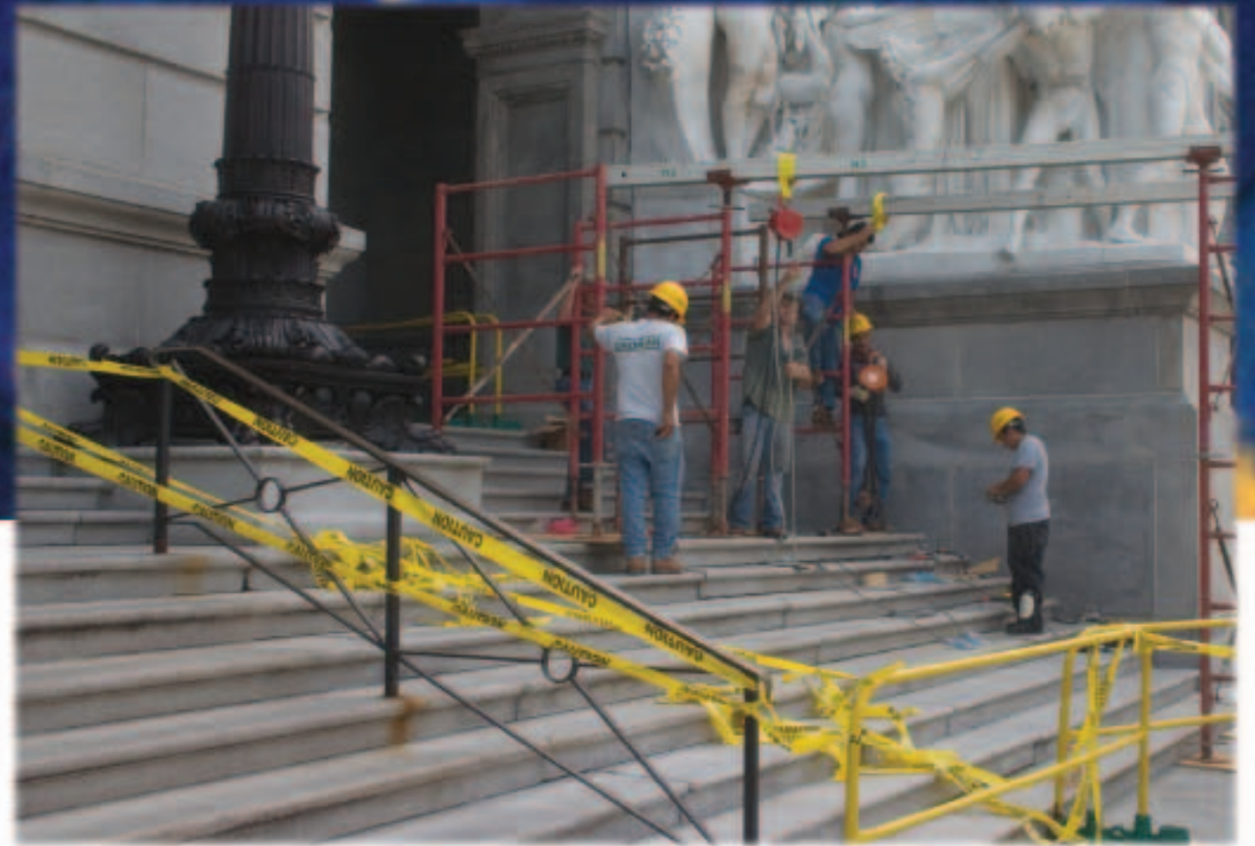
WORKERS ERECT SCAFFOLDING TO HOIST TREADS FROM THE CAPITOL'S WEST STEPS
