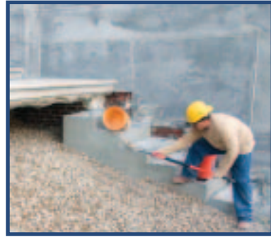
INSTALLATION OF RIVER ROCK
