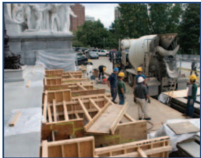
FORMS ERECTED FOR NEW CONCRETE PIERS
