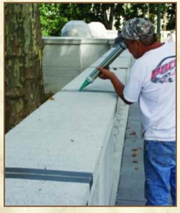
Repointing Failed Joint in Balustrade
