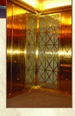
The design pattern for the elev ators' interior brass panels was adapted based on elements from the 1906 elevators. In addition, the larger rotunda elevators to the west have been fitted with translucent corner panels, which let in natural light
