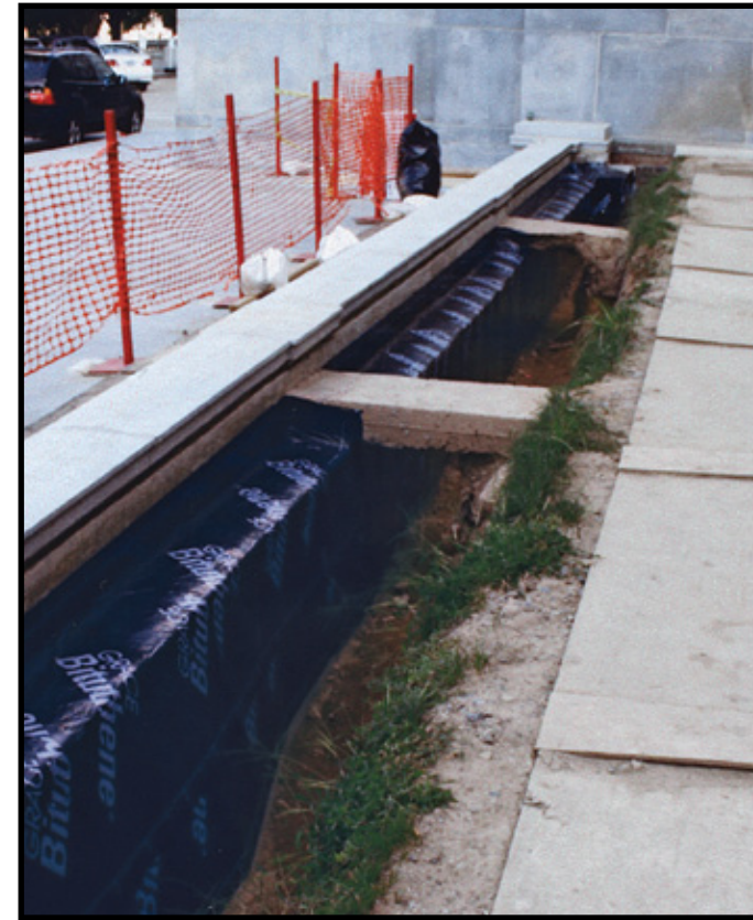
BITUTHENE 4000 MEMBRANE APPLICATION AT THE NORTH HYPHEN WALL
