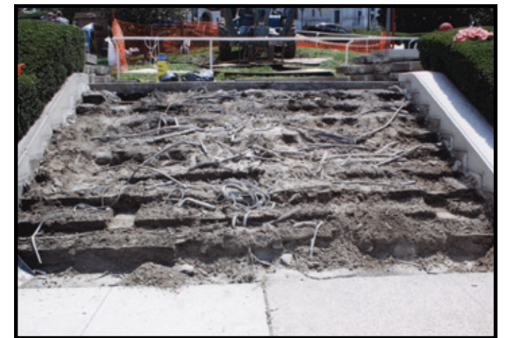
VIEW OF UNDERLYING SUPPORT FOLLOWING REMOVAL OF ALL GRANITE TREADS.
