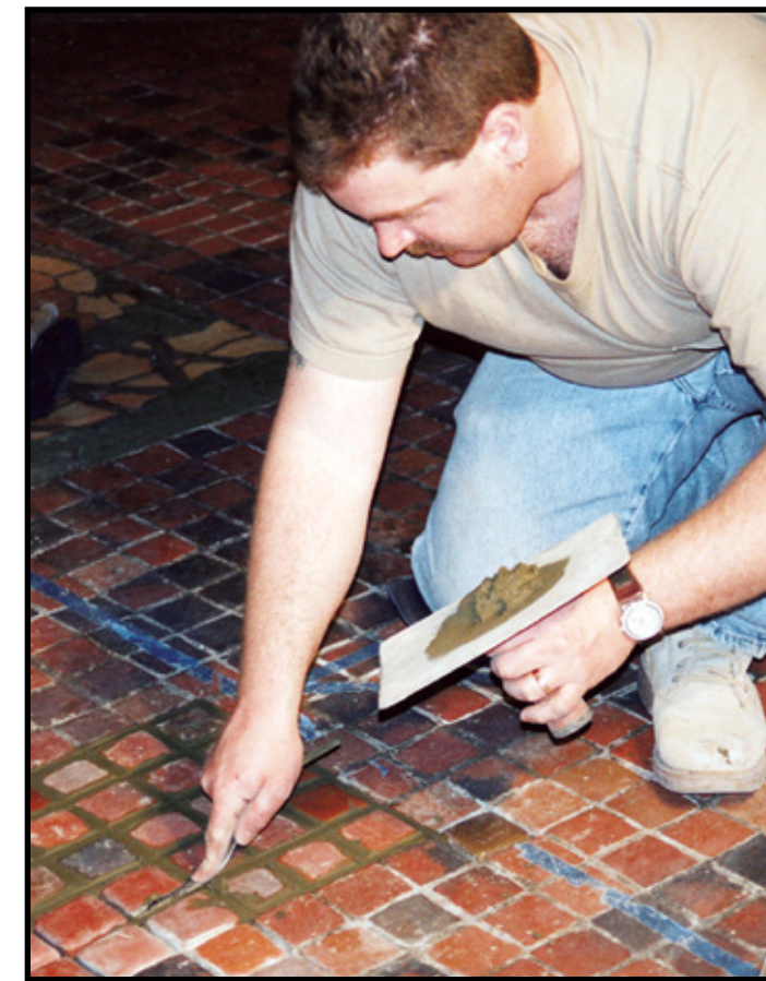
TECHNICIAN PAT MCBRIDE GROUTS REPLACEMENT TILES.
