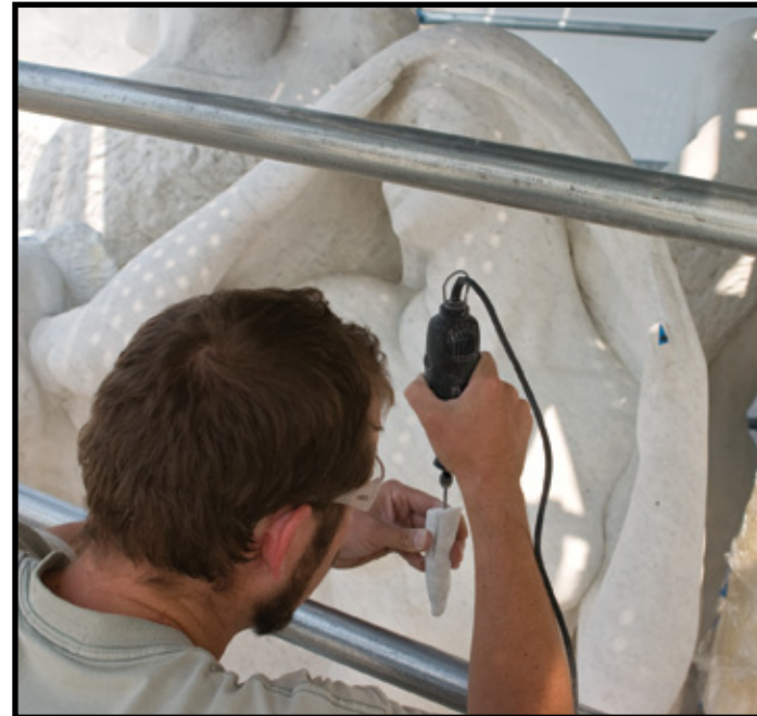
SCULPTOR INSTALLING DUTCHMAN REPAIR
