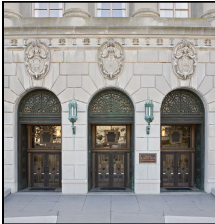
SOUTH OFFICE BUILDING, FIRST FLOOR NORTH ENTRANCE.
