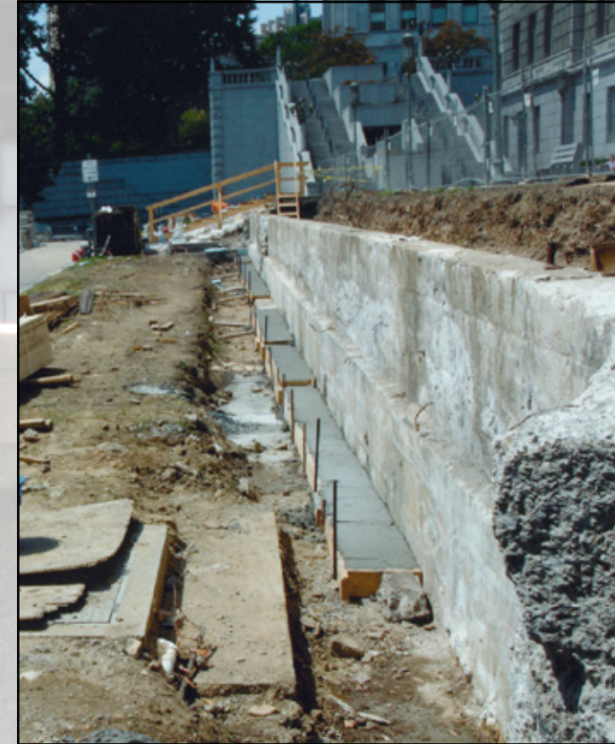
View of existing foundation wall and new additional foundations.
