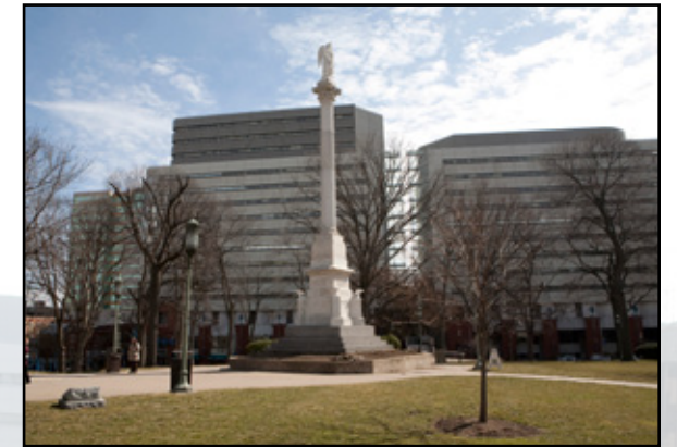
View of the Mexican War Monument area prior to the rehabilitation of South Capitol Park
