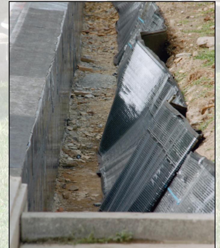
Detail of initial waterproofing fabric in the excavated area.
