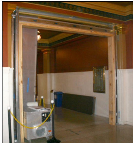
Installation of double-leaf doors
