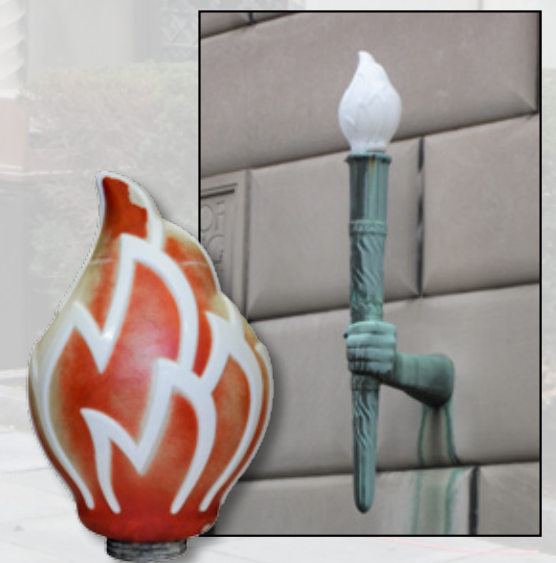
Left: Flame globe prior to cleaning Right: Installed flame globe outside Forum Building entrance
