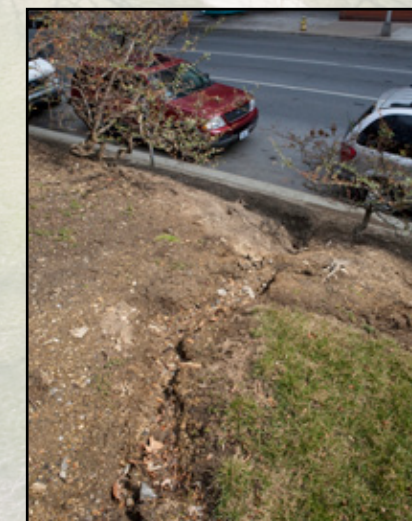
Eroded bank due to stormwater runoff
