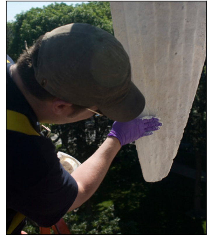
Application of lime shelter coat on wings of Angel.
