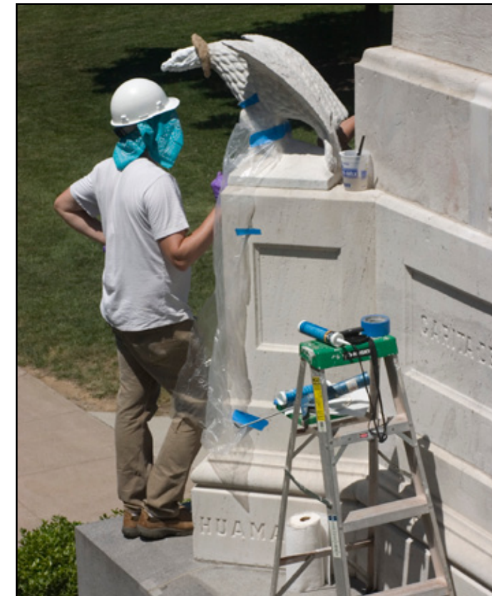
Mold being prepared for Dutchman repairs.
