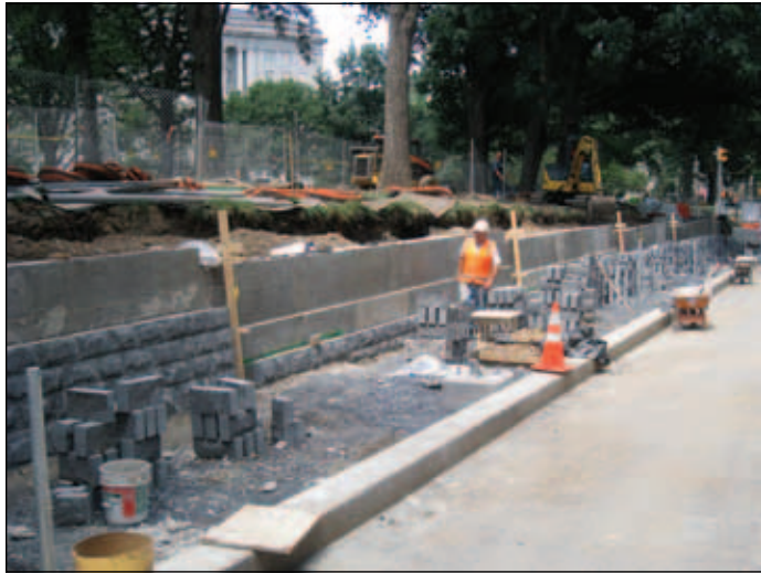
Installing granite veneer on Walnut Street retaining wall
