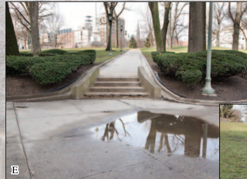
E. Ponding water on sidewalk F. Heaving sidewalk and erosion G. Walnut Street embankment looking east H. Old park bench I. Clogged stormwater inlet
