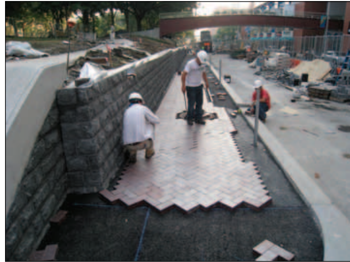
Installing brick sidewalk along Walnut Street
