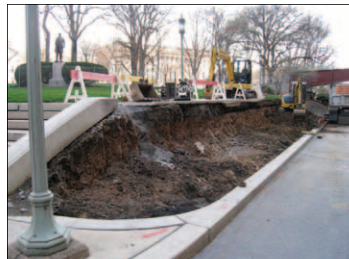
Excavating Walnut Street Sidewalk
