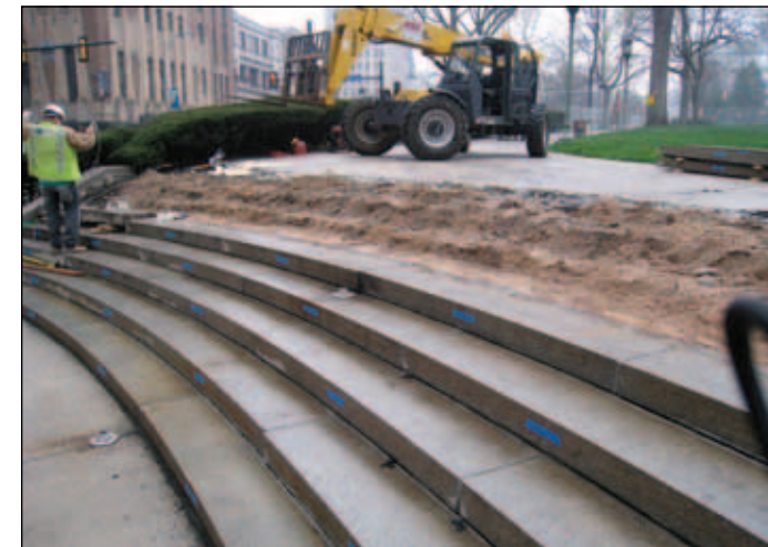
Removal of steps at Third and Walnut Streets
