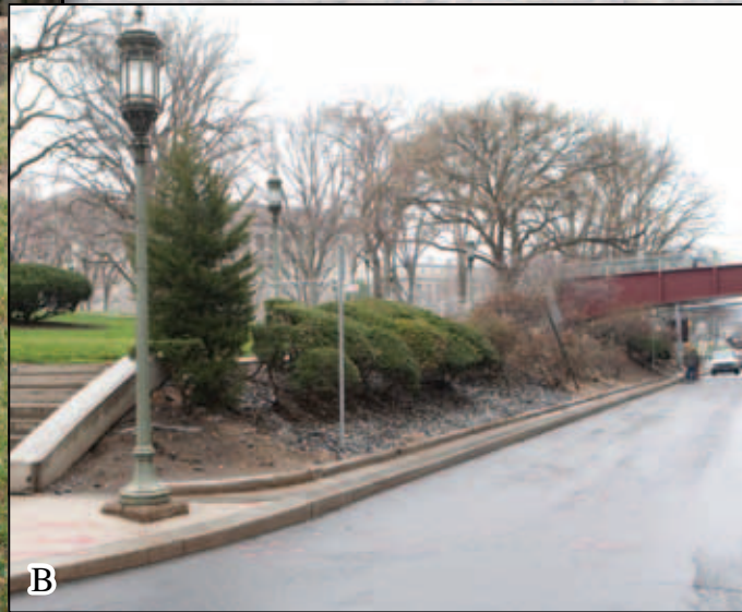
A. Walnut Street embankment looking west B. Walnut Street looking east C. Erosion D. Erosion
