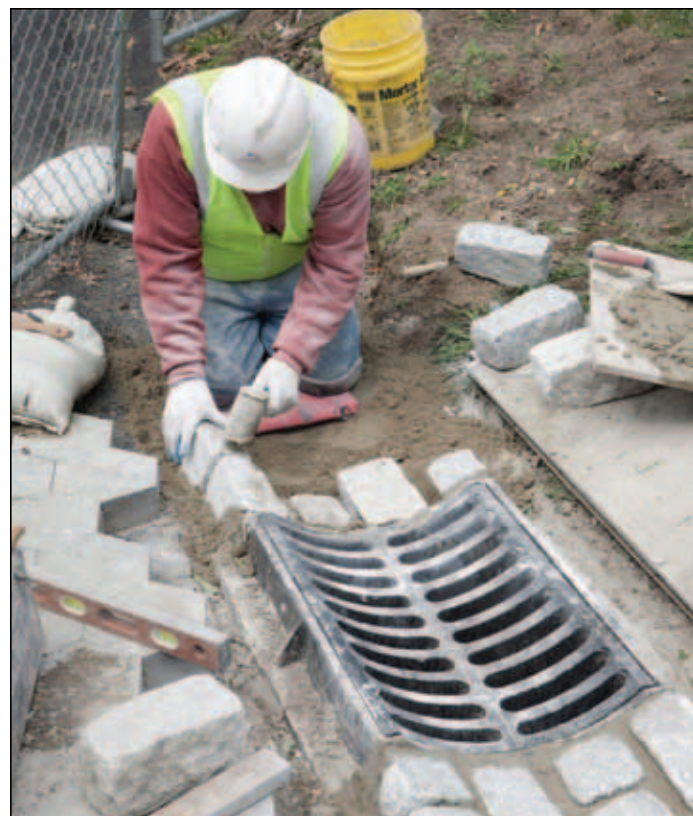
Installing cobblestone gutters
