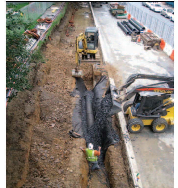
Installation of stone and filter fabric around drainage pipe
