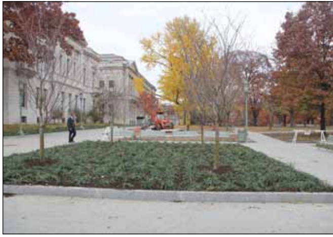
Hartranft Plaza with installed asphalt pavers and landscaping
