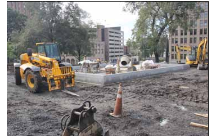
Hartranft Plaza after demolition with partially installed granite planting area
