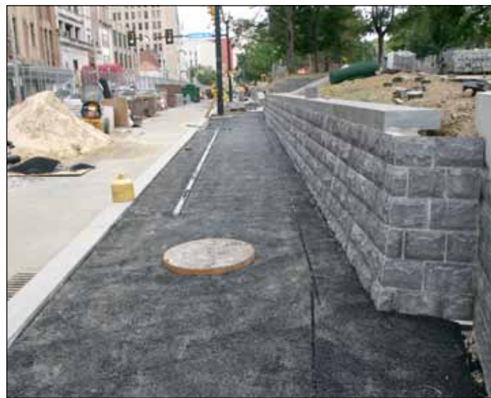
Sidewalk with asphalt bed and granite curb along Third Street
