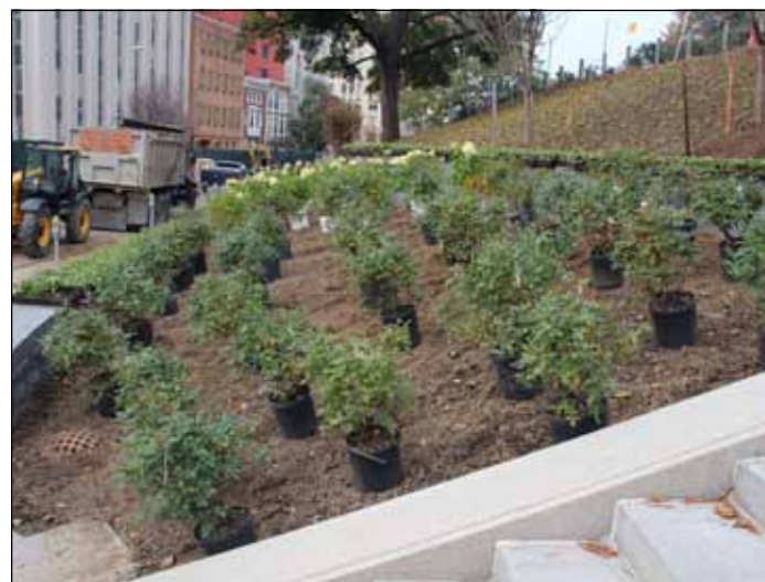
Planting area to the north of the Locust Street steps
