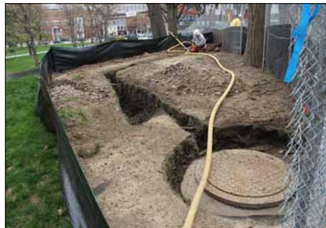
Exposed roots using SSAT excavation
