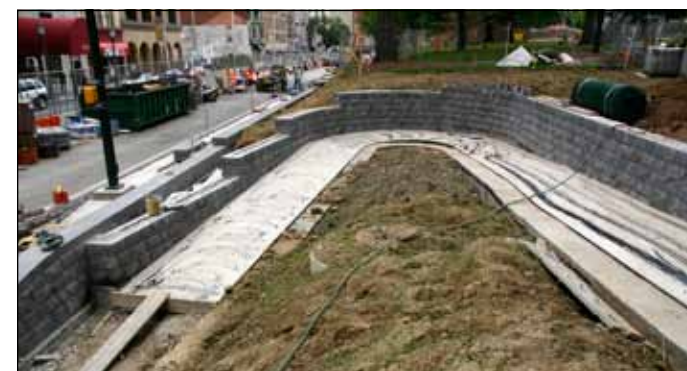
Handicap ramp with poured concrete base, retaining wall and granite facing
