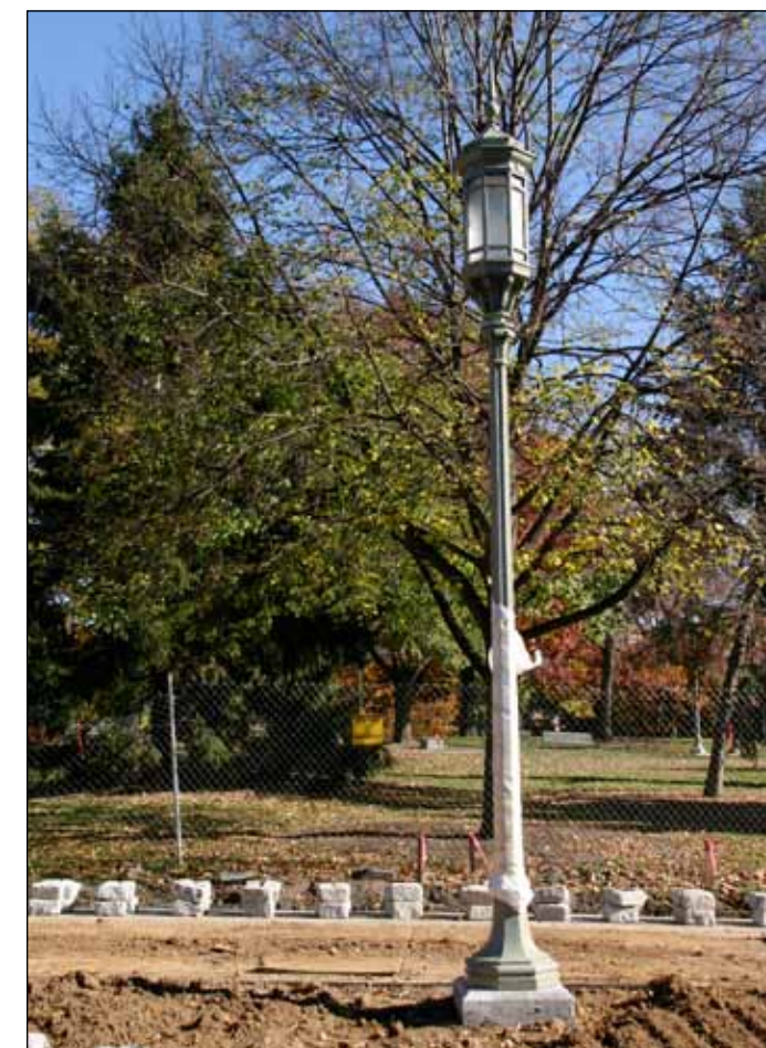
Restored light fixture along interior park path
