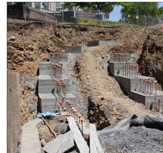
Excavated area with cheekwall footers at Pine Street steps
