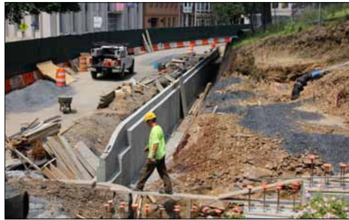
Excavated bank along Third Street with footers and concrete wall
