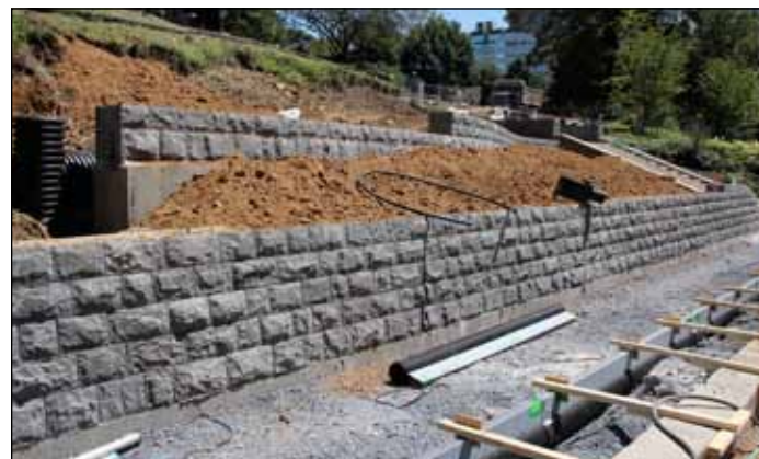
Retaining walls with installed granite facing
