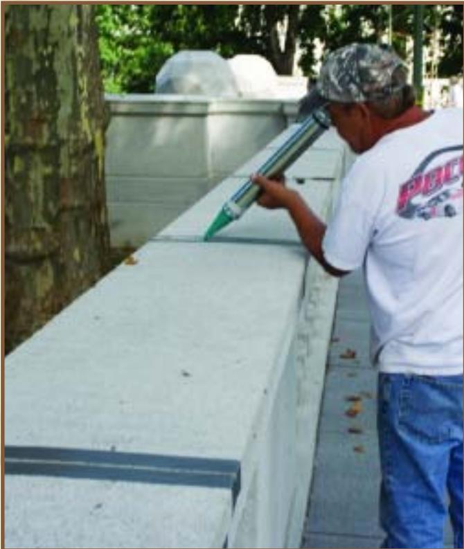
*Repointing Failed Joint in Balustrade*
