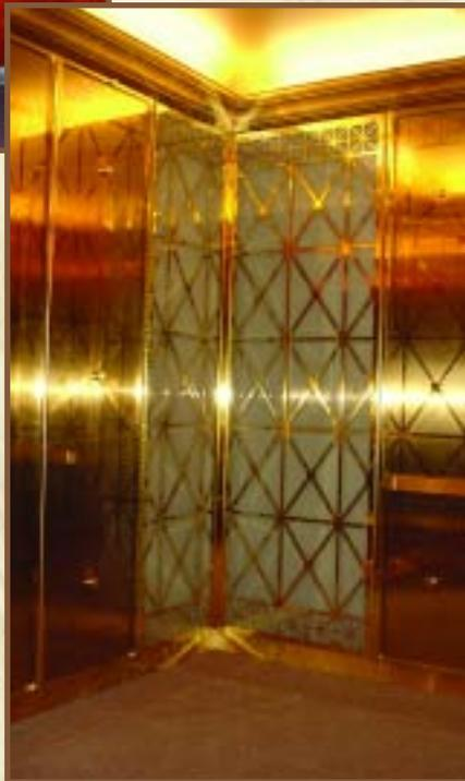
The design pattern for the elevators' interior brass panels was adapted based on elements from the 1906 elevators. In addition, the larger rotunda elevators to the west have been fitted with translucent corner panels, which let in natural light
