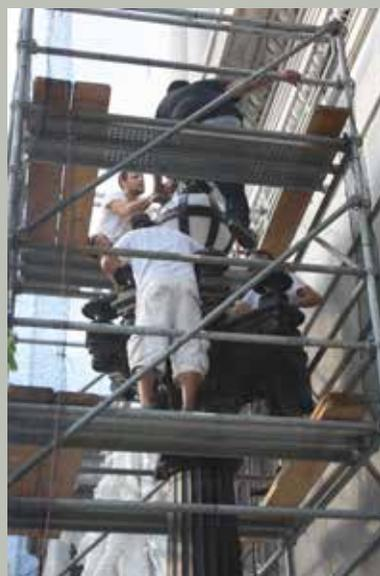
of the fixtures, which had become sun-bleached over time. Several new bronze castings made to replicate the original lanterns, as they were installed in 1906, were attached at the top of the fixtures. Before replacement any cracks, breaks and repairs to the original glass were noted and replacement glass may become
