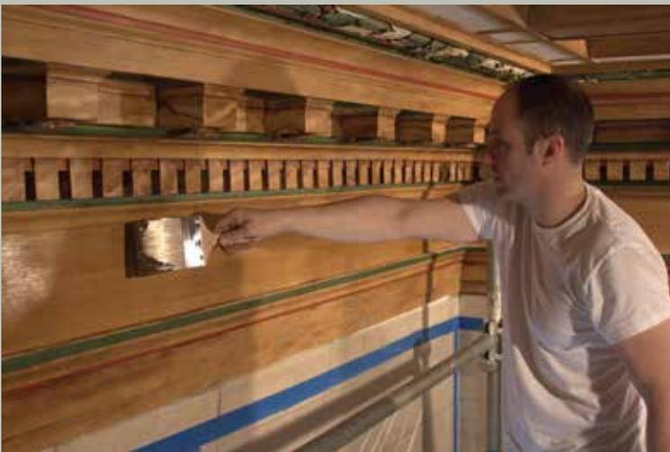
sample boards before being painted to match the original 1922 glazes as much as possible. Upon completion the entire ceiling was inspected, photographically documented and dusted and vacuumed.
