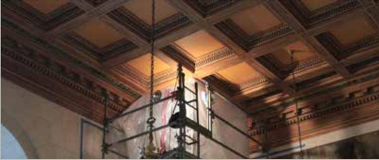
Over the course of fall and winter 2013 the committee undertook repair of the damaged plaster cornice in the Plaza Level Lobby of the Irvis Office Building. Scaffolding was erected so conservators could document the existing conditions of the damaged plaster. After documentation, damaged and loose areas of plaster were removed. A 6 mil plastic bubble was constructed around the damage to properly abate any lead during the project and workers wore Tyvek suits and respirators during
