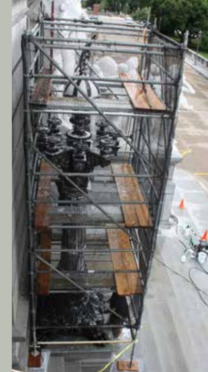
The lanterns under the portico had some weather damage to the initial wax coating flaking and deteriorating over time. The historic glass was removed, cleaned and placed in storage, while the lanterns were first vacuumed and then cleaned with a solution and soft brushes and allowed to dry overnight. The lanterns were then treated using heated wax which was reapplied to areas of loss, especially the west-facing façade
