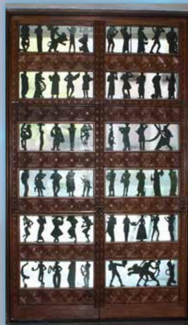
were complete, a patina was reapplied to each door using a ferric nitrate and water solution. The door jambs were also cleaned and treated, and a patina re-applied. Lastly, the threshold anchors and closers were re-aligned before each door set was re-installed. The restoration of the Lawrie doors shows just how beautifully-designed and ornate the Art Deco Forum Auditorium was, both inside and out, upon its completion in 1931. Ongoing cyclical maintenance of this
